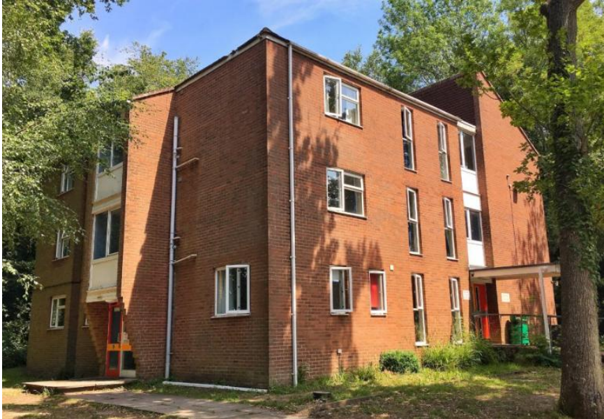
Heald House: a 3-floor, 90 bed block in 2,3,4 and 6 bunk bed rooms. There is an en-suite leaders' room on each floor. Wifi available.
